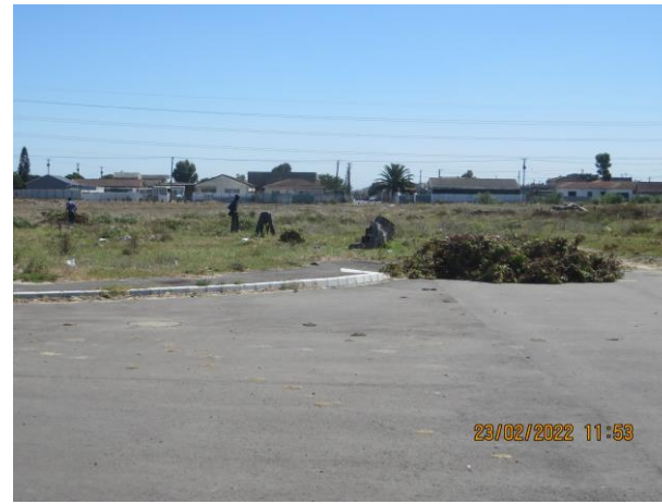
Ongoing vegetation clearing over Phase 5 and 6
